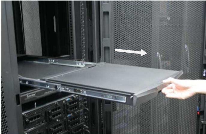
**Figure 4.** Sliding out the LCD keyboard drawer by pressing the carry handle button first.
